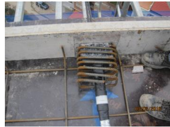
CASE II : TWO LAYERS OF TOP REBAR
